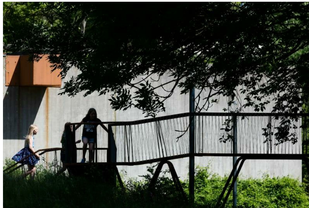
The Loop Gladsaxe, Denmark. Holscher & Nordberg Architecture and Planning
