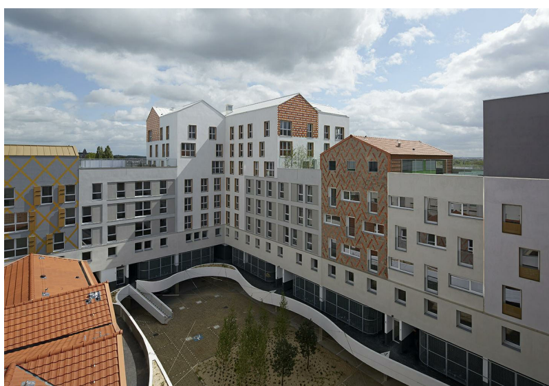
Pontoise Housing. Architects Atelier du Pont. Foto Frédéric Delange
