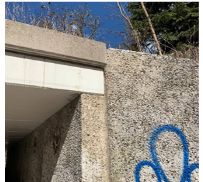
Befintlig situation. (Bild, Bjerking)
